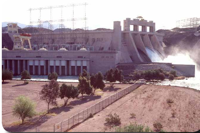
Bureau of Reclamation’s Davis Dam (left above) and the DeCew II Generating Station operated by Ontario Power Generation (right).
